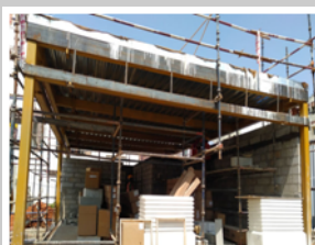
STEEL STRUCTURE BUILDING
