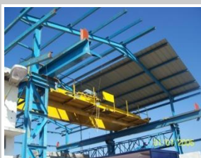
STEEL STRUCTURE AND ROOF DISMANTLING
