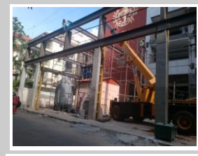
STEEL STRUCTURE BUILDING EXTENSION
