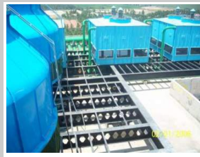
COOLING TOWER PLATFORM
