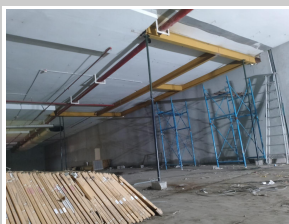
CONCRETE SLAB STRENGTHENING
